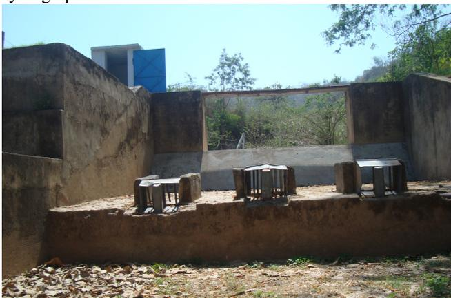
**Fig. 4: Runoff gauging station at the outlet of the watershed.**
