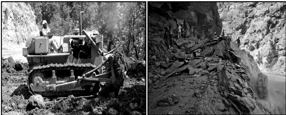
Fig. 6: Construction and blasting on the banks of Mandakini and Alaknanda rivers (Source: http://www.downtoearth.org.in/content/uttarakhand-floods-disaster-human-induced )
