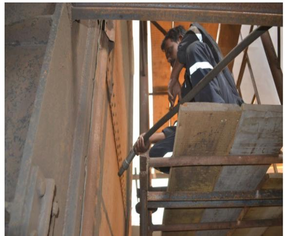
**Fig. 2: Preparation of Gate Surface using CI Grit Blasting**
