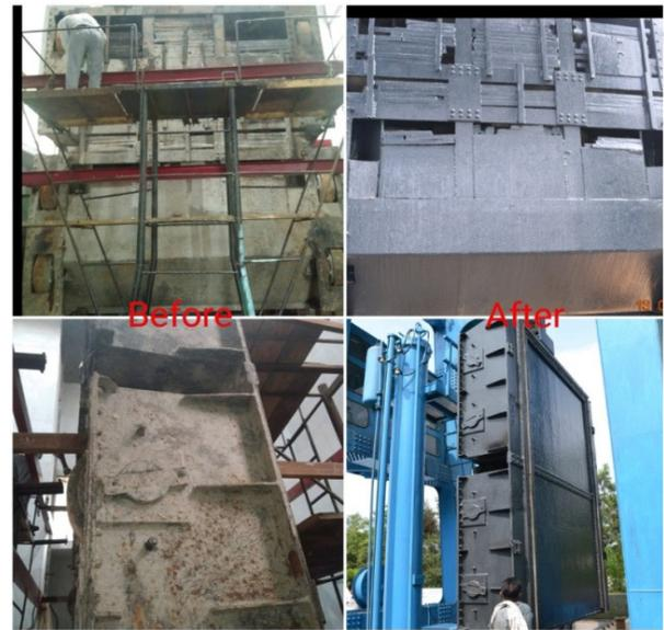
**Fig.4: Comparison for Gate surface before and after treatment with ceramic paint.**
