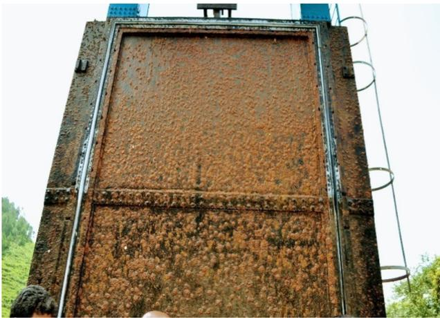
**Fig.1: Condition of Gate treated with CA-50 Paint when taken out for annual repair**
