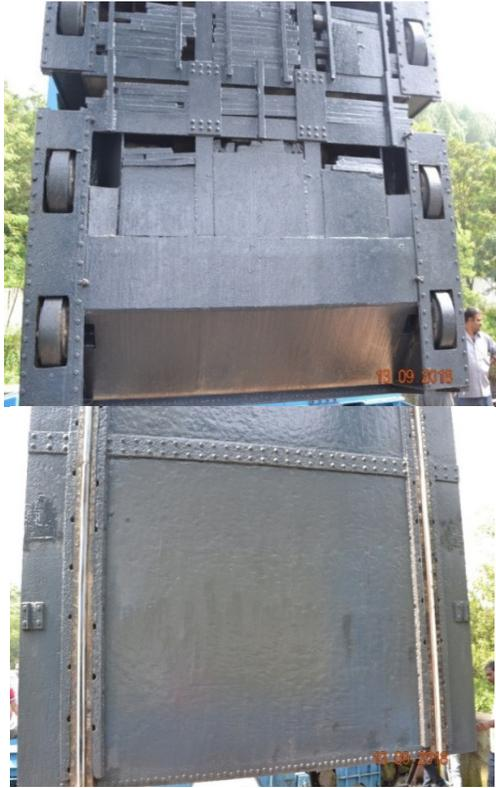
**Fig.3 Gate surface ( u/s & d/s) after application of Ceramic coating and has given glossy and shiny look.**
